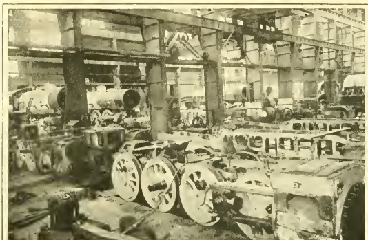
Erecting shop, locomotive works, Schenectady
